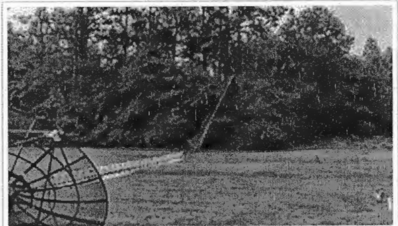
This radio tower collapsed on Wednesday in Kosciusko, Mississippi after a tree fell onto a guy wire.
