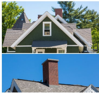
APPLICATION: Roof Attached Chimney | LOCATION: Saratoga Springs, New York DESCRIPTION: 3' wide, 8' tall, 2' deep
