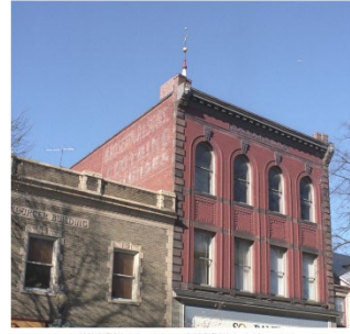
APPLICATION: Colored Chimney | LOCATION: Annapolis, Maryland DESCRIPTION: 2' wide, 7' tall, 4' deep
