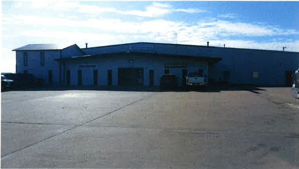
Existing Facility facing North
